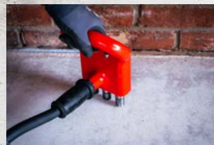
Reducing Levels on Concrete
